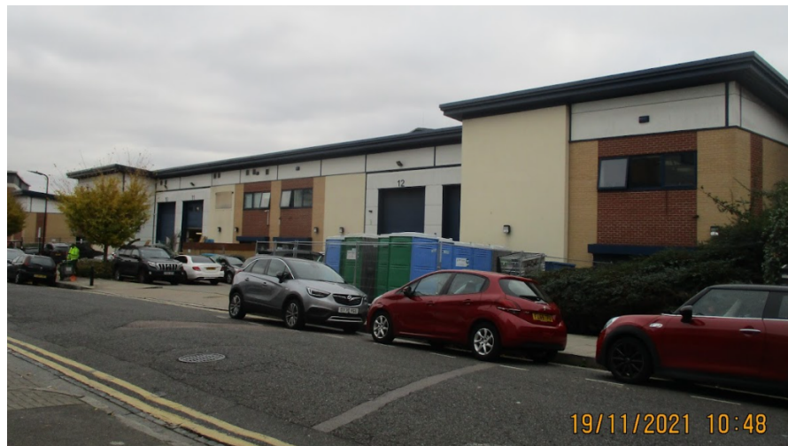
Figure 1 Existing Building on Site
